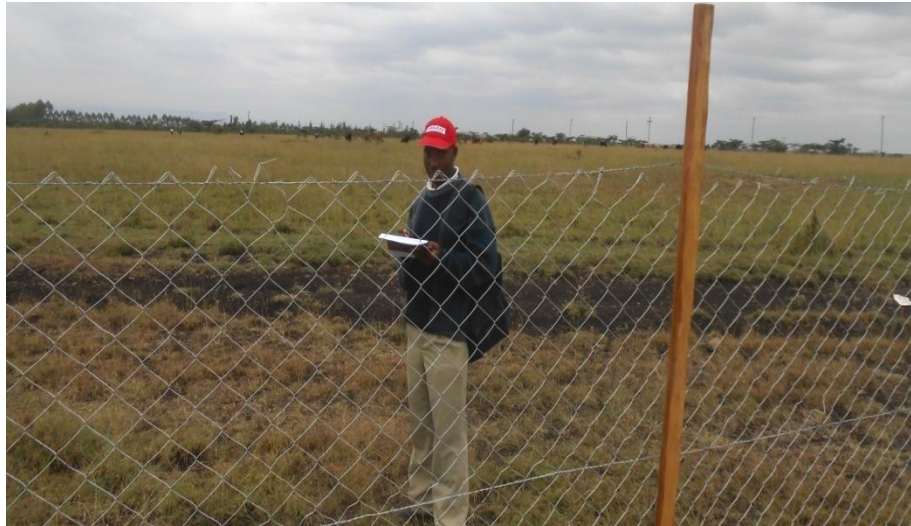
Figure 2 . This chain-link fence was under construction during study period.
